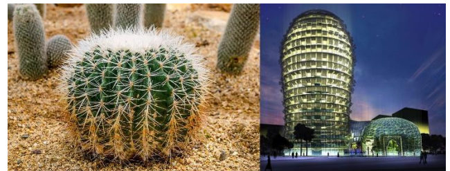
Figure 8. Qatar's giant cactus the building is covered from its top to its bottom with shades that resemble the spines in the cactus plant.
